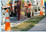
Cutting a trench for the fiber conduit.
